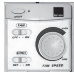
**Note:** On days of high humidity the fan may be operated without the pump. For ventilation only, turn the Cool switch OFF which turns the pump OFF.
